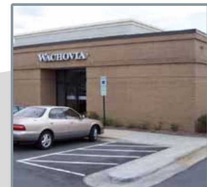
Wachovia @ North Hills, Raleigh, NC Before panelized wall systems
