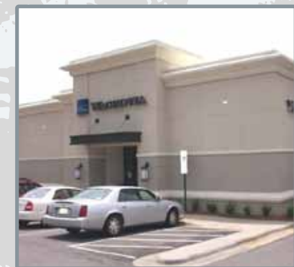
Wachovia at North Hills, Raleigh, NC After panelized wall systems
